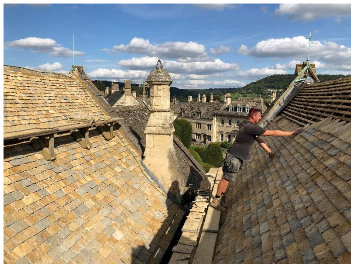
Re-roofing of the organ chamber/vicar's vestry north slope
