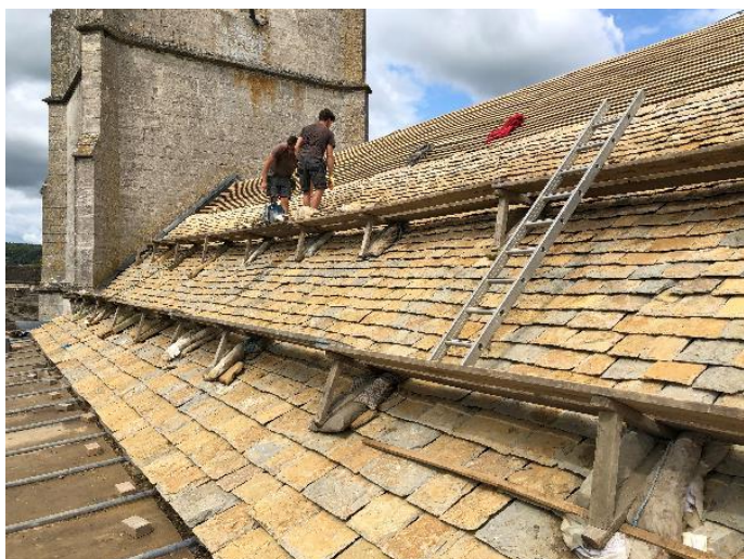
Re-roofing the north slope of the nave
